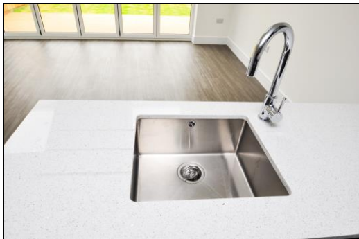
Under-mounted sink, granite worktops
